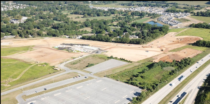
Easton, PA | 500,000 SF Flex | Under Construction
