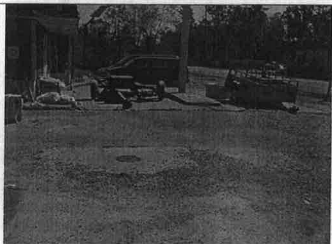
5-003559 Kirby 76 10/16/03 Location of underground storage tanks
