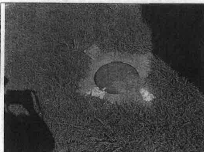
5-003559 Kirby 76 10/16/03 Groundwater Monitoring Well
