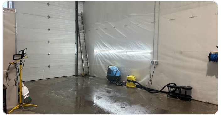
Open, heated drive-in bay with ~12' overhead door
