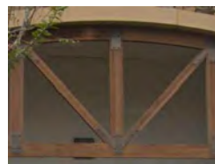
10 WOOD ARCHWAY BROWN TEAK WOOD REF. MATCH EXISTING SHOPPING CENTER REF. MATCH EXISTING SHOPPING CENTER COLOR CUSTOM BROWN SEE 3/A-400
