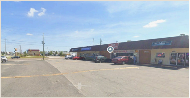
Full strip-center elevation — units 5004 — 5016 along US-19.
