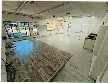
Previous Nail Salon, plumbing set up.
