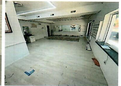
View from front door, laminate floors.
