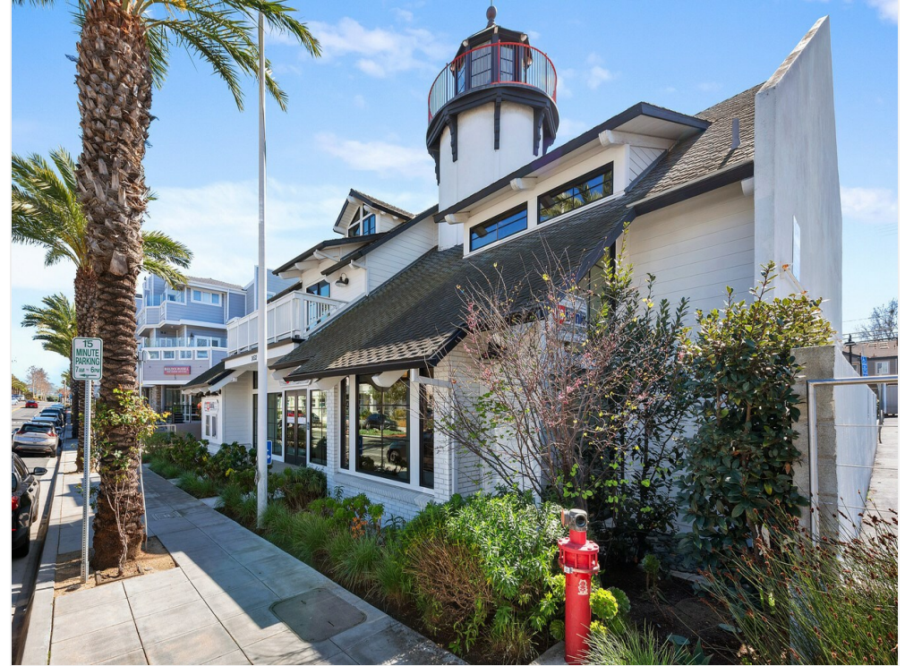
Front of Building
