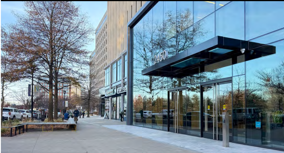
LOOKING SOUTH ALONG THE CRYSTAL DRIVE STREETSCAPE
