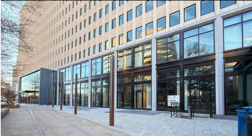
LOOKING SOUTH ALONG THE CRYSTAL DRIVE STREETSCAPE
