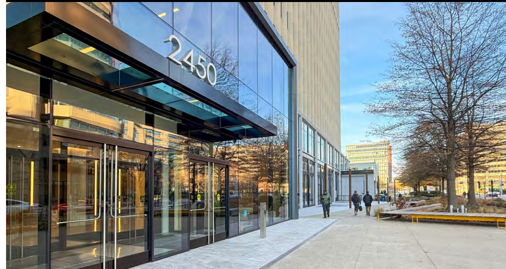
LOOKING NORTH ALONG THE CRYSTAL DRIVE STREETSCAPE
