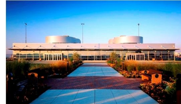
Rickenbacker International Airport
