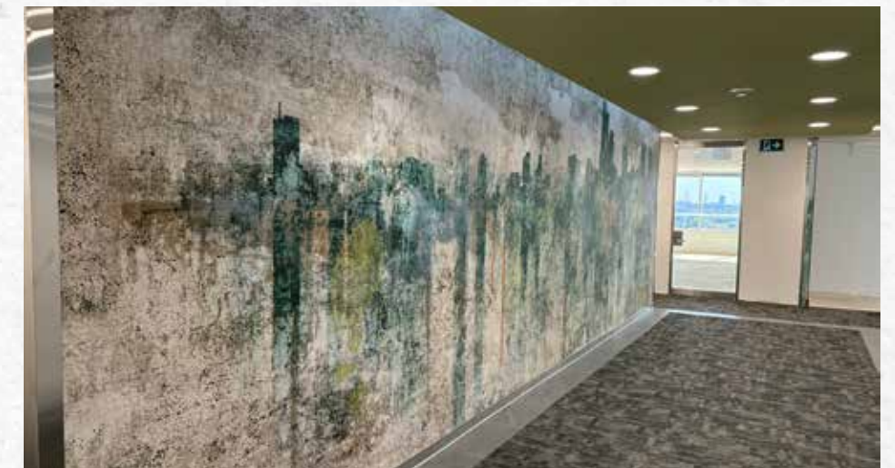
5TH FLOOR HALLWAY ELEVATOR
