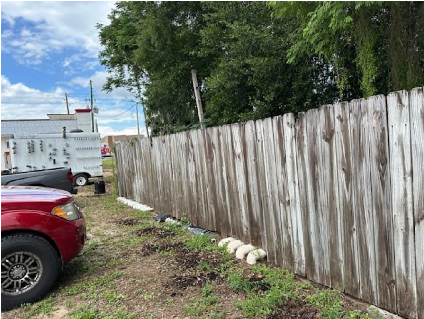
Outside Equipment Compound, West Side, with Remedial Equipment Trailer in Left Background, Facing NNE
