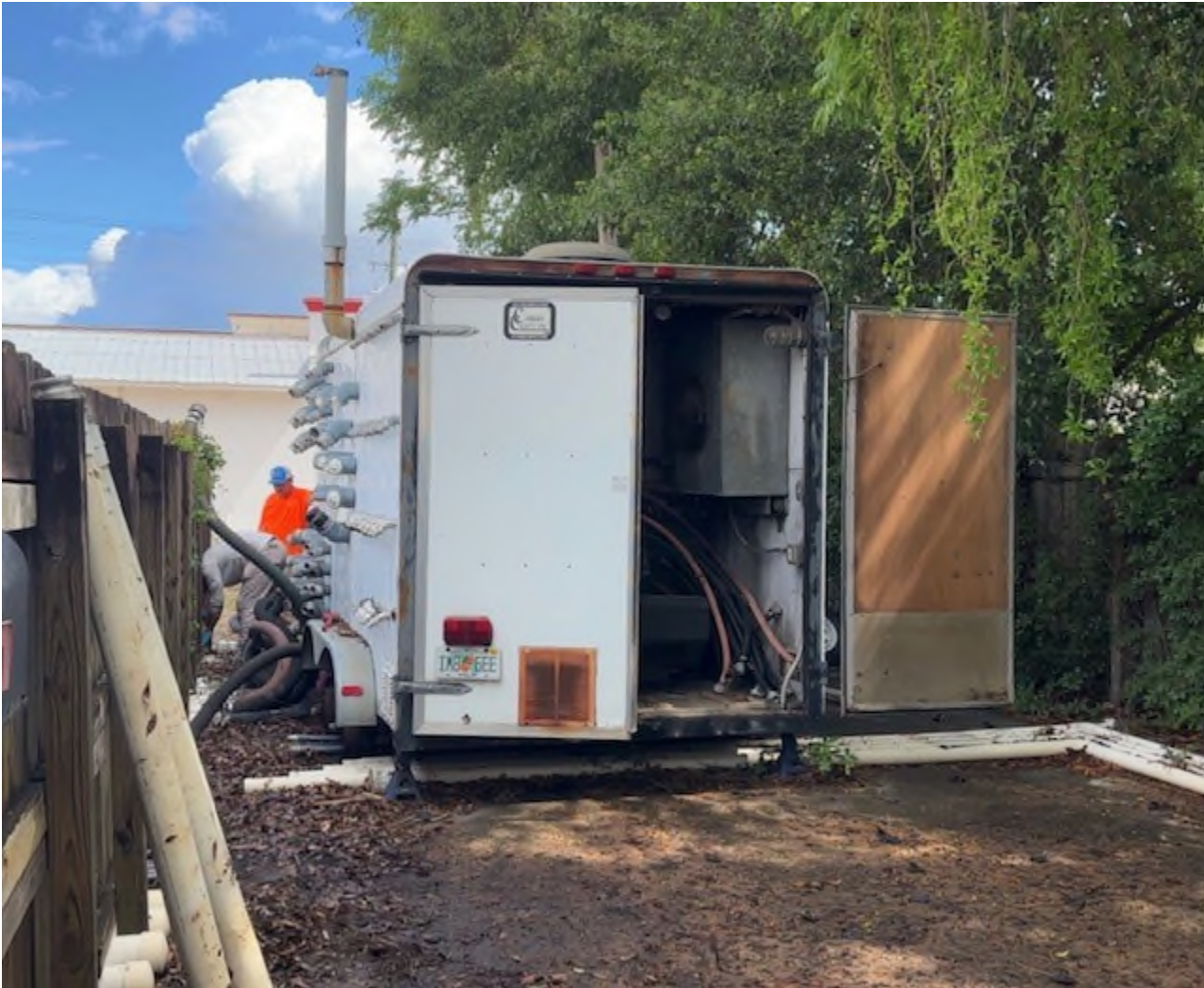
Disconnecting Hoses and Conduit from System Trailer, Facing North
