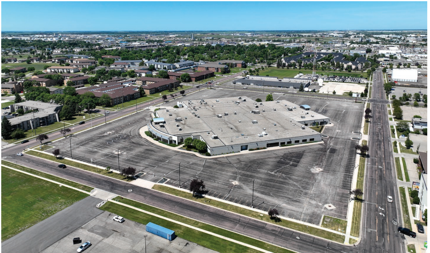
LOOKING TO THE NORTHWEST
