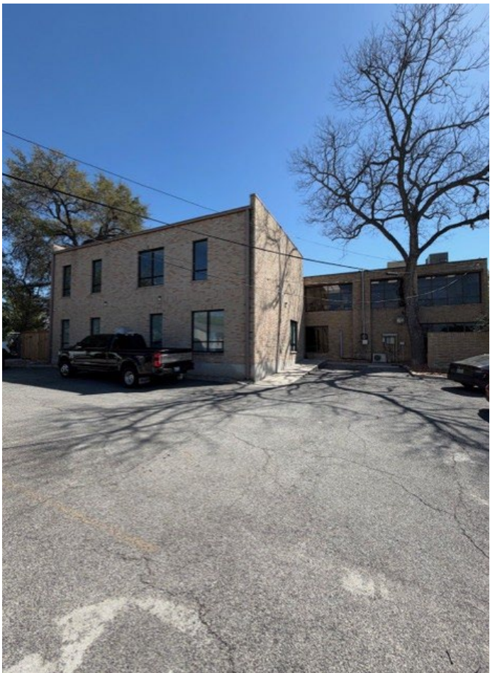
Rear / parking court view
