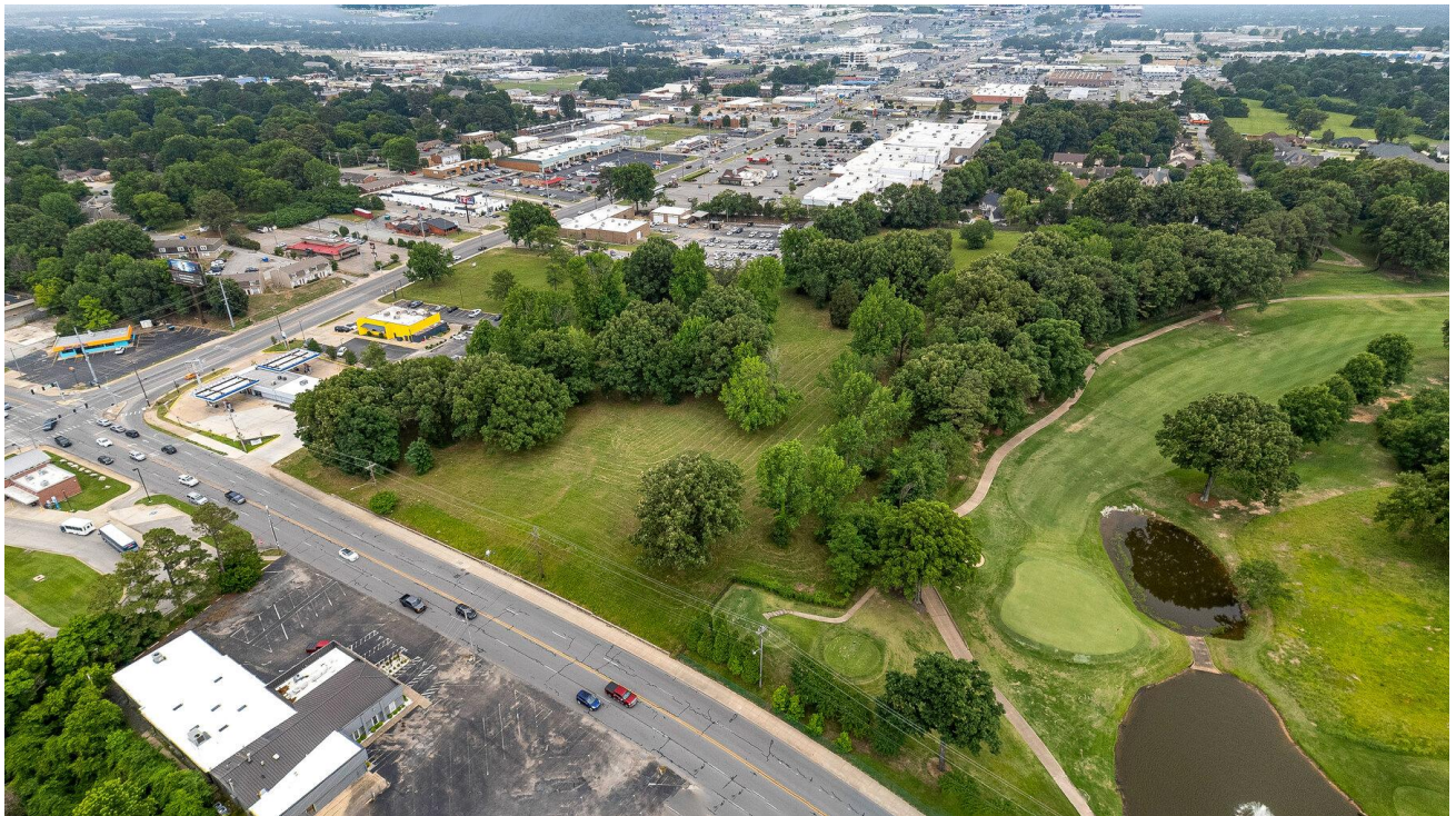
Drone aerial showing the property's relationship to the Jonesboro Country Club golf course fairway (right), the transit corridor, and surrounding commercial development.
