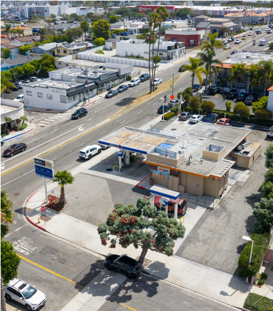
Aerial — subject property at Manhattan Beach Blvd
