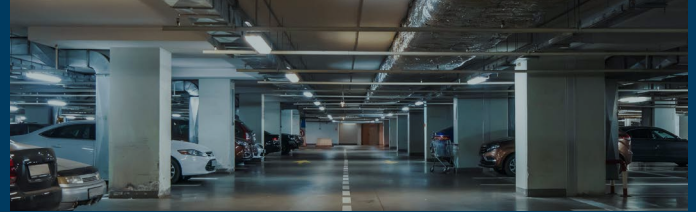
Four levels of underground parking with automated entry/exit system serviced by two dedicated parking elevators. Daily car detailing and car wash service.
