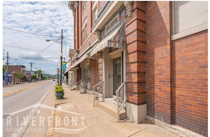
West Southern Avenue streetscape and storefront entries.
