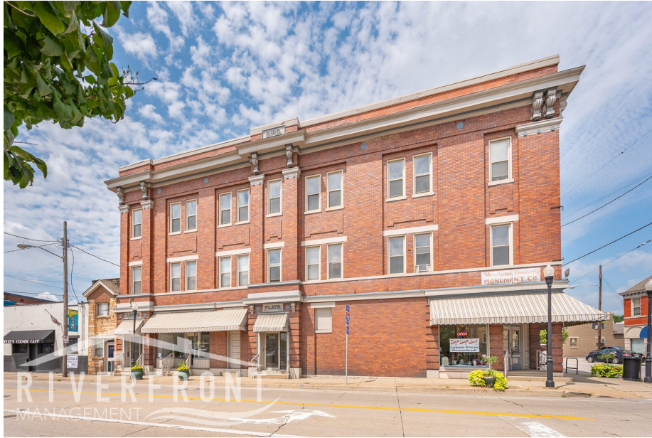
Primary façade on Winston Avenue — striped awnings, masonry cornice, and the historic BYRD nameplate.
