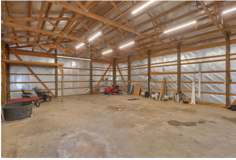
Shop Interior — Concrete Floor & 220 Power
