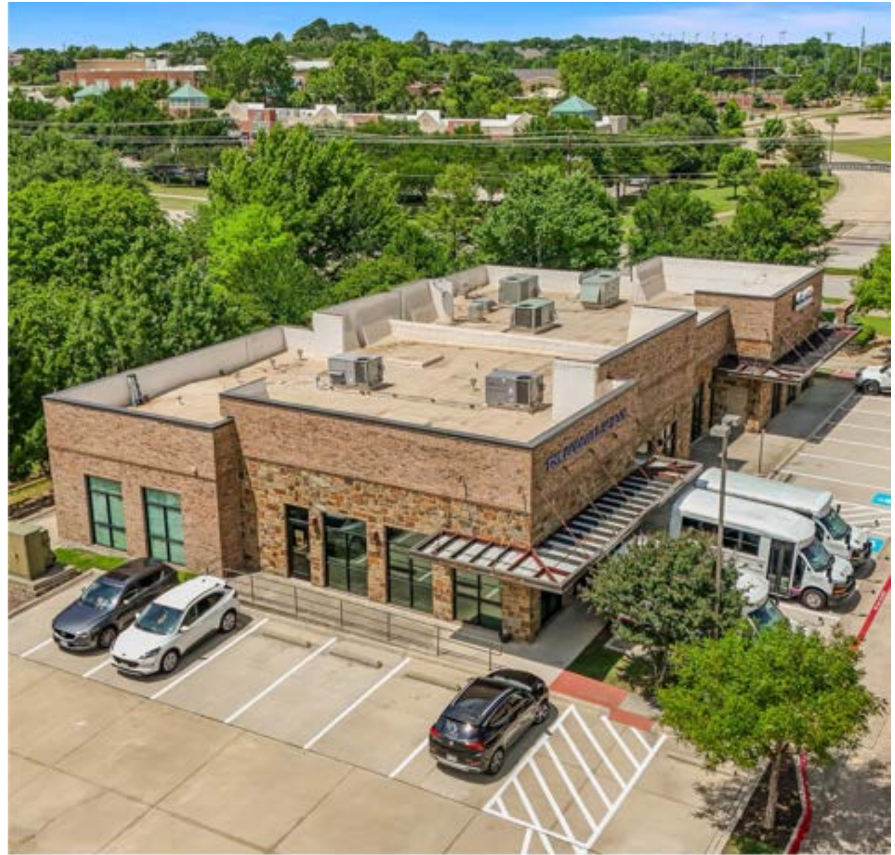
EXTERIOR · 445 W SOUTHLAKE BLVD
