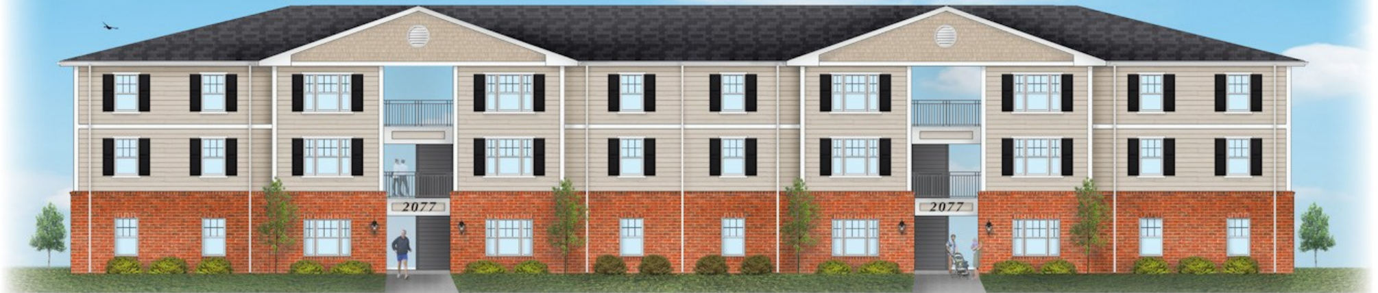
Entitled 84-Unit Trinbrook Apartment Site
