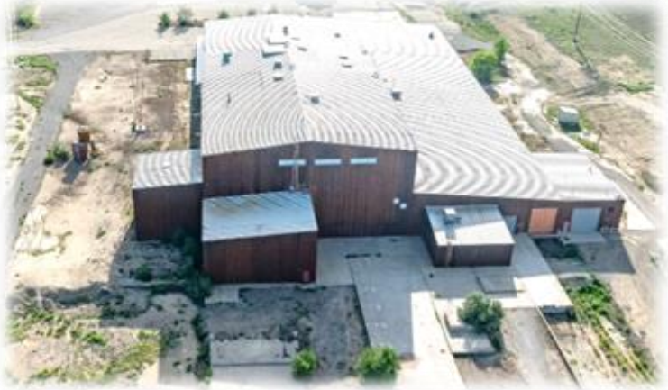
View of Facility facing East/Back of Building
