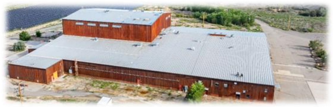
View of Facility facing South
