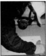
Wear protective clothing and a respirator when removing walls that may contain lead.
