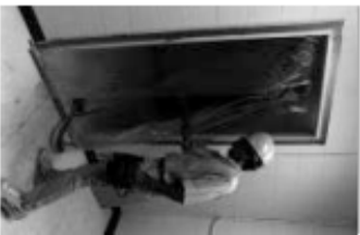
Close off entryways with an airtock.
