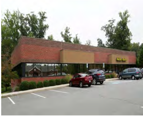
Townsend Office Park 1955 Emancipation Hwy Fredericksburg, VA 22401
