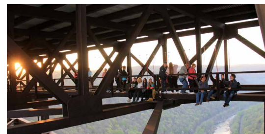
New River Gorge Bridge Walk
