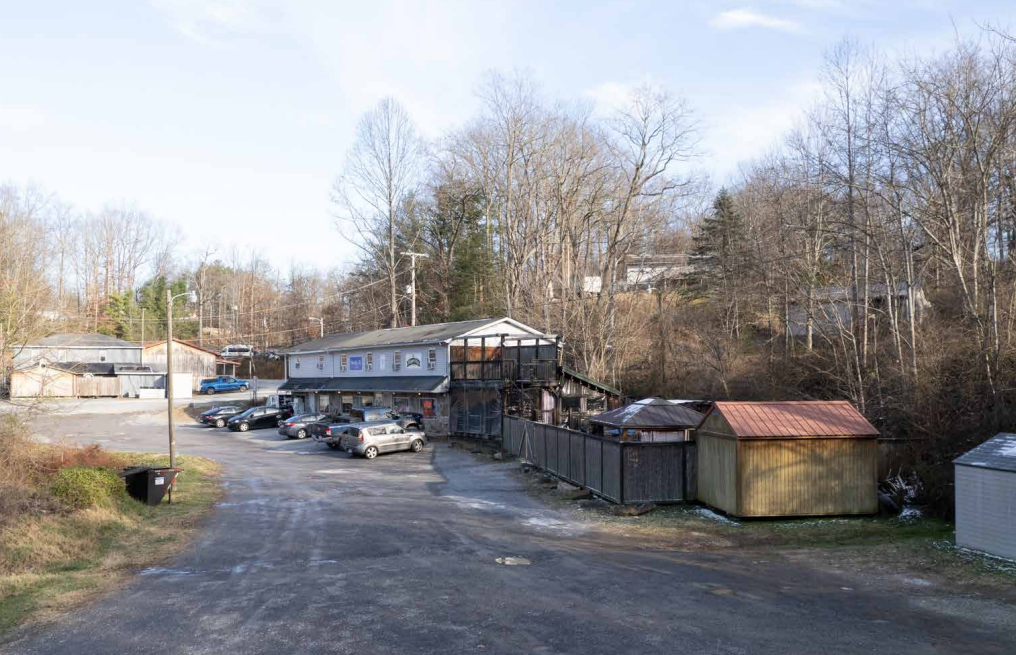
Exterior Side View of the Building.
