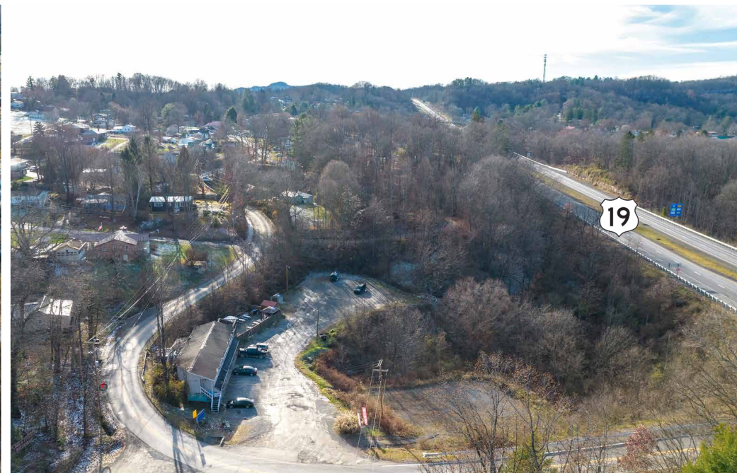
Aerial Facing South.
