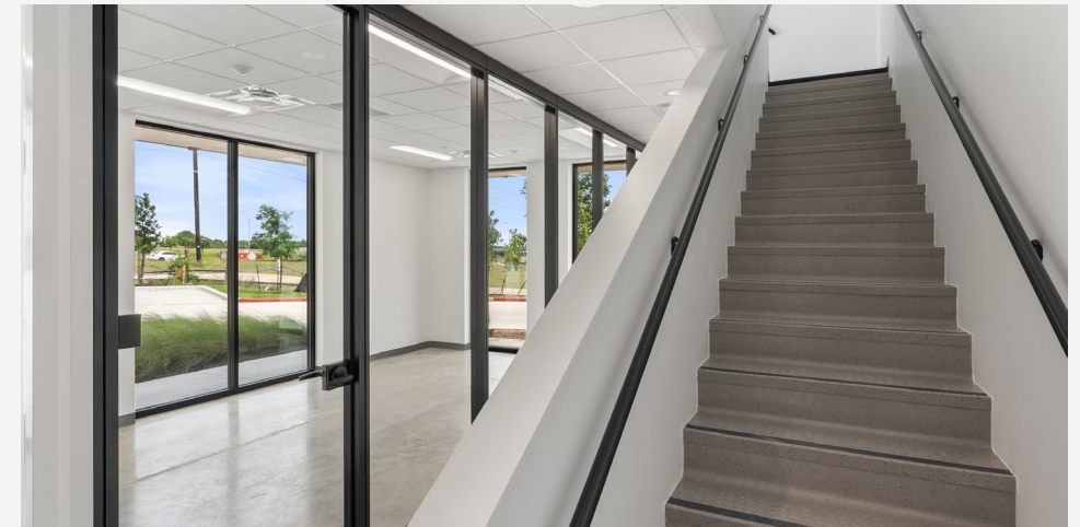
Interior stair connecting Level 1 and Level 2
