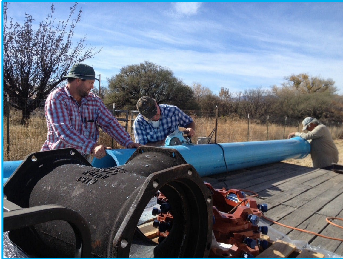
Building the 12 Inch Pipe riser insert
