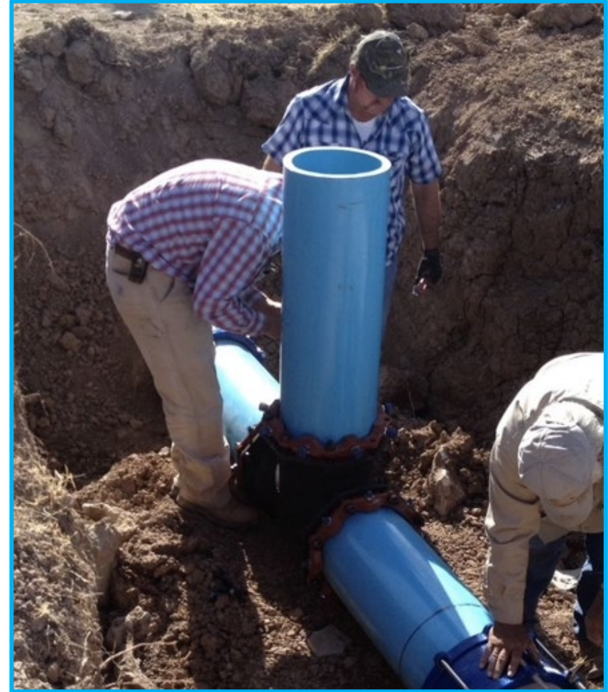
Connecting assembly & riser
