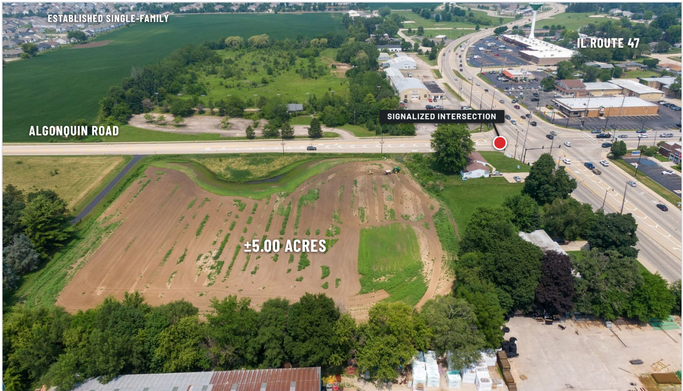
Looking north across the property. Algonquin Road forms the north boundary; IL Route 47 and the signalized intersection are at right.
