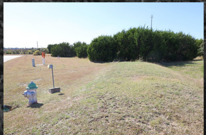
Image 6. General site conditions and utility infrastructure from neighboring property facing south
