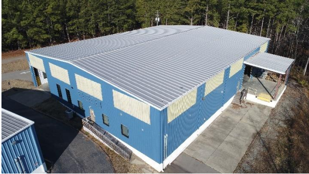
Dock Side - Warehouse Exterior
