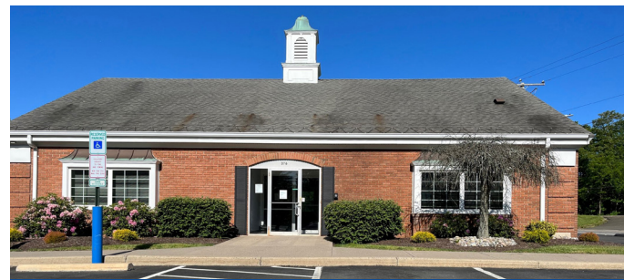
376 Main Street ±3,328 sf office/retail space
