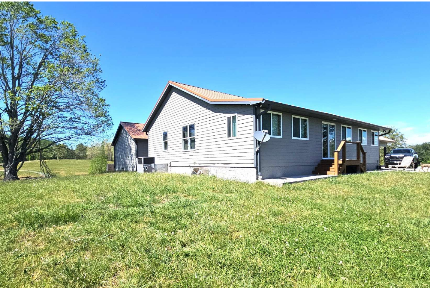
REAR DWELLING – VIEWING NW
