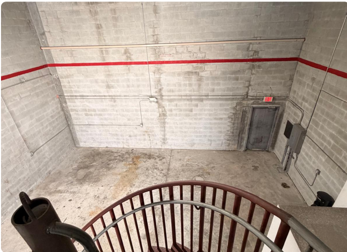
Access to Mezzanine
