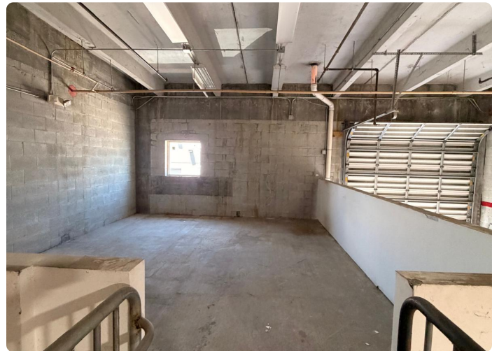
200 SF Concrete Mezzanine
