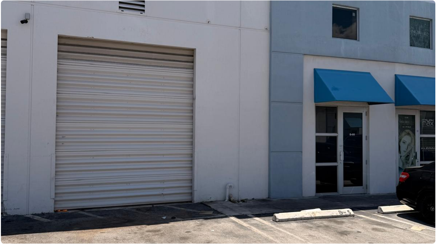
Front Exterior & Loading Door
