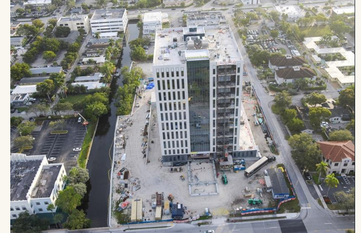
SUBJECT & COURTHOUSE SITE — TWO BLOCKS
