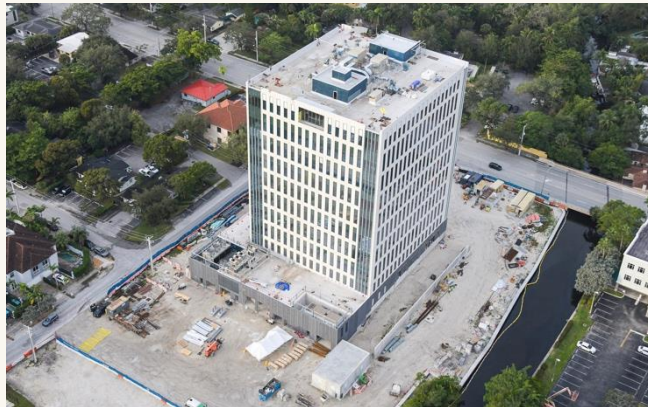
COURTHOUSE UNDER CONSTRUCTION, 2026
