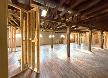
UPPER FLOOR — HEAVY TIMBER POST AND BEAM
