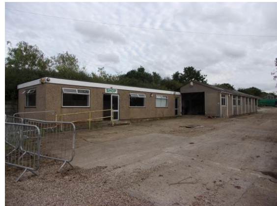
Office/unit. Original photo.
