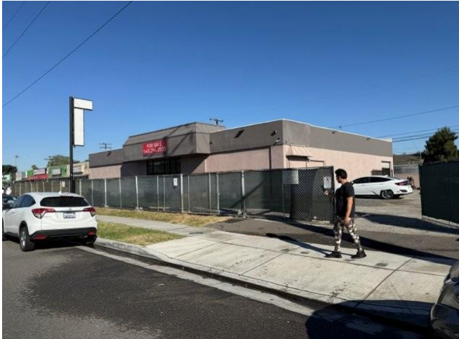
Southern elevation from Carson Street
