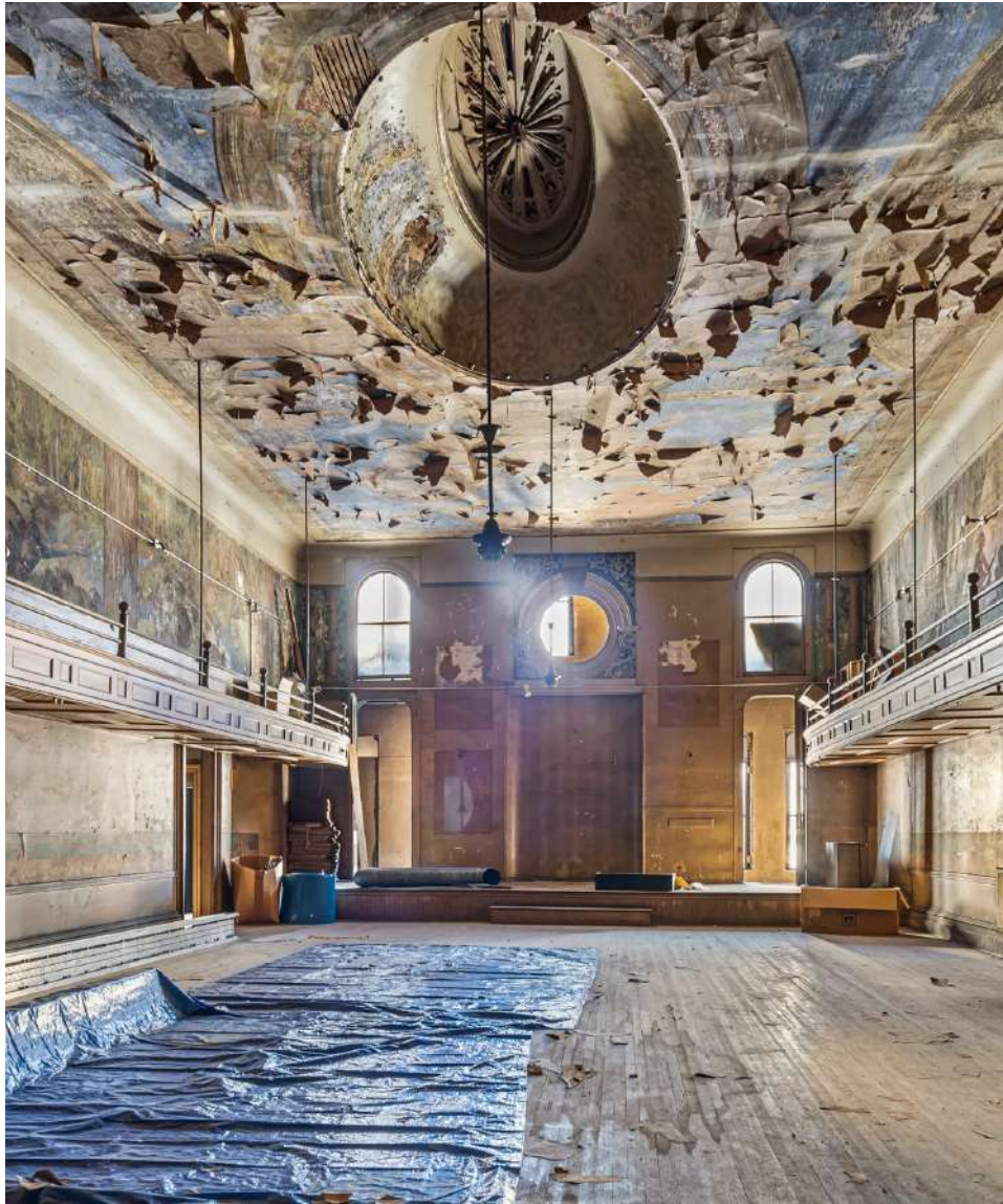
Historic Wamsutta Lodge Hall with Original Murals, Wraparound Balcony and Ornamental Ceiling Dome.
