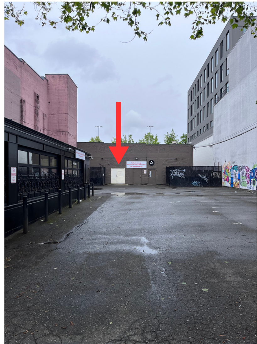
Above: Rear Delivery Entrance, Marked With Red Arrow
