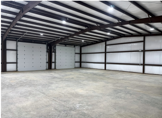
Warehouse interior — open span, LED lighting, insulated walls
