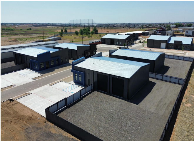
Building yard and fenced storage area
