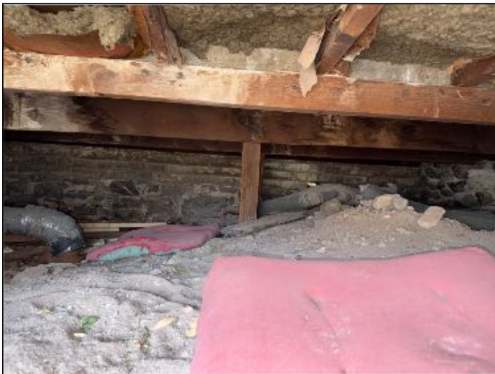
View of crawlspace
