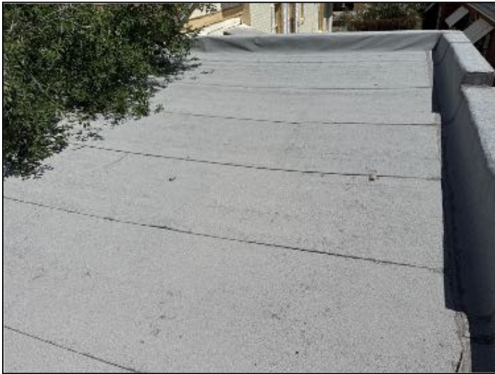
View of roof top material
