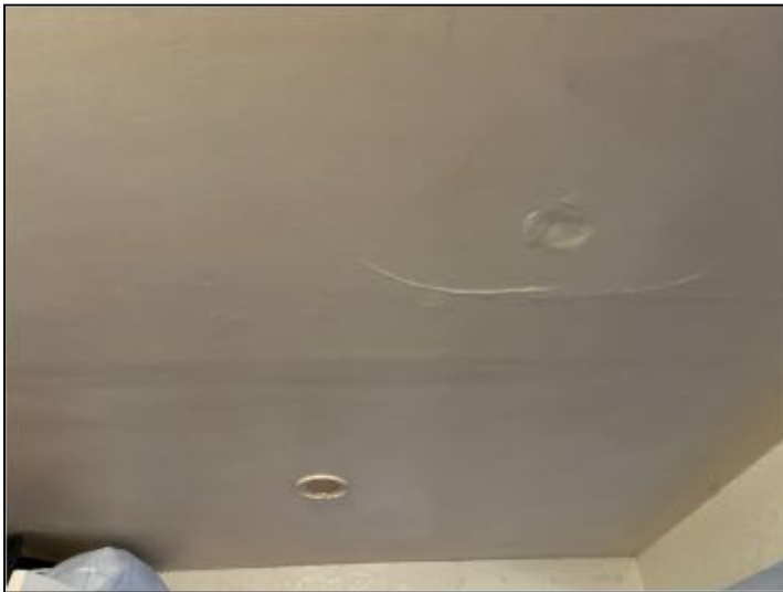
SAFETY CONCERN: Carbon detectors were missing in hallways . Recommend correction as to allow proper function: all units
