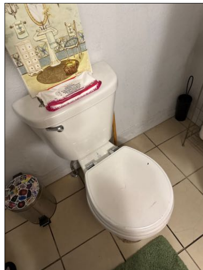
MAINTENANCE:Commode seemed to be loose from base. Recommend correction as to prevent water seeping onto floor: unit 3
