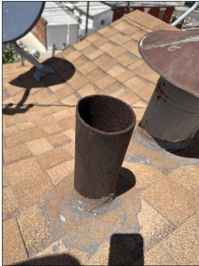
A sewer scope inspection was performed on the main laterals drain lines at the time of the inspection. One or more deficiencies were noted in the accompanying report, including channeling of pipes, standing water . Further evaluation and or repairs by a plumber are advised.
