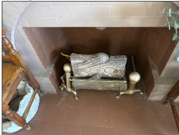
Fireplace gas flow was functional as need be: unit 3
