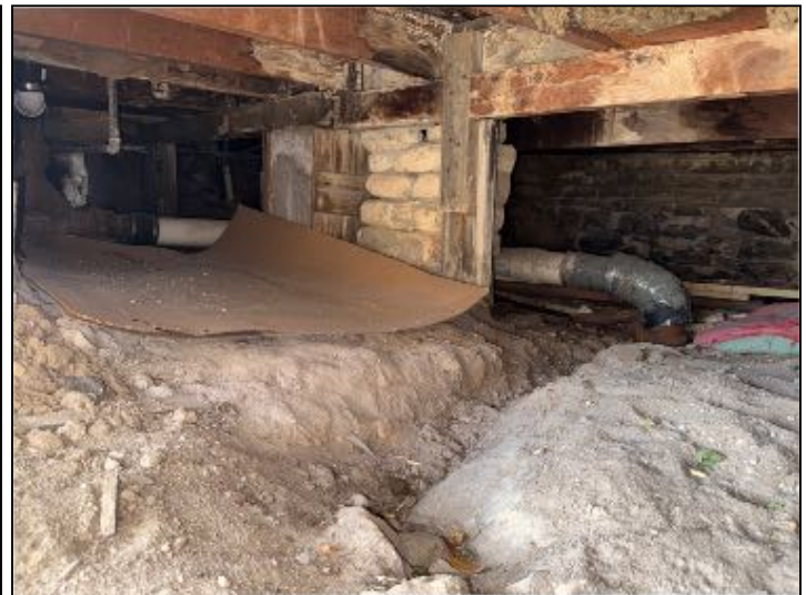
View of crawlspace
