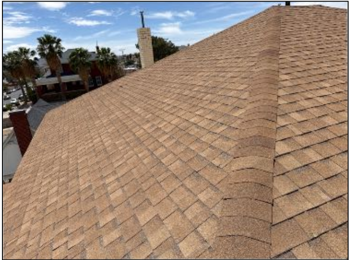
View of roof top material
