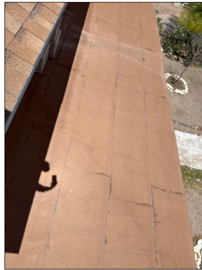
View of roof top material
