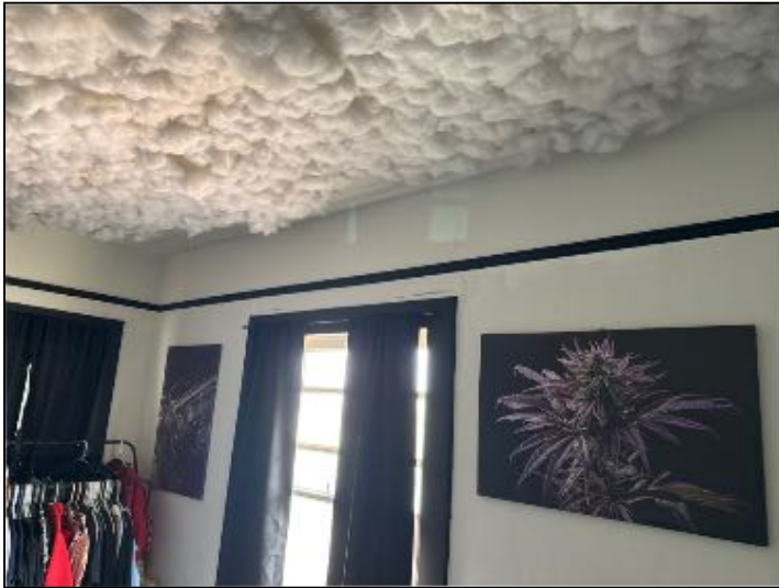
View of cracks in walls of unit 1
