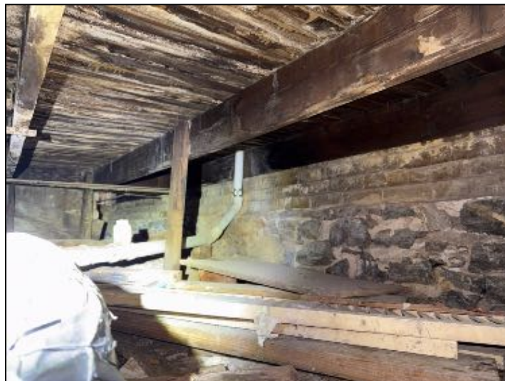
View of crawl space wall
