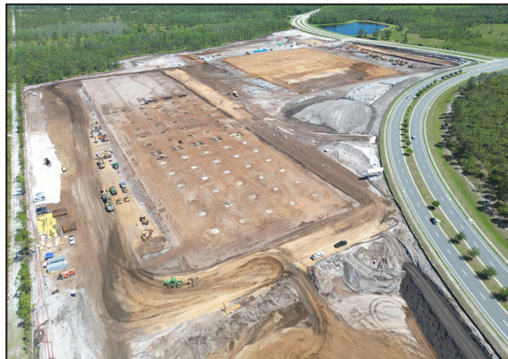
CONSTRUCTION PROGRESS - PREPPING PADS
