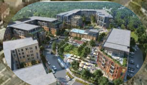
Westchester Crossing Boston Post Rd 975 Residential Units Hotel - Mixed Use *In Construction
