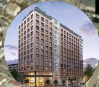
155 Irving Ave 181 Residential Units
