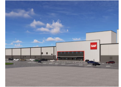
GAF Newton $350M | Under Construction
