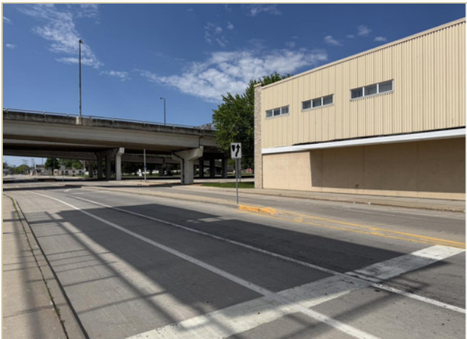
CORNER AT THE MASON STREET OVERPASS — ARTERIAL VISIBILITY
