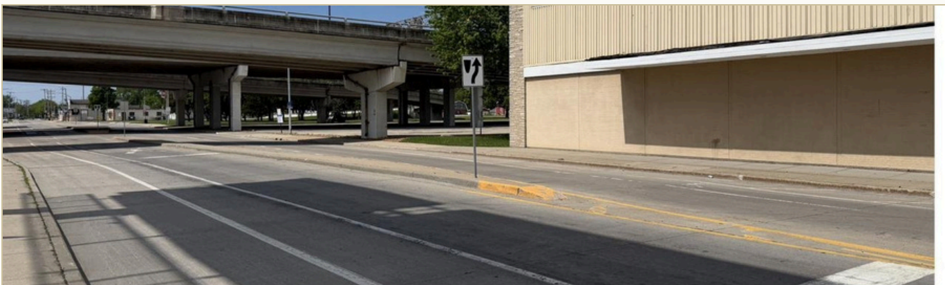
SUBJECT AT THE MASON STREET OVERPASS — HIGH-VISIBILITY HARD CORNER
