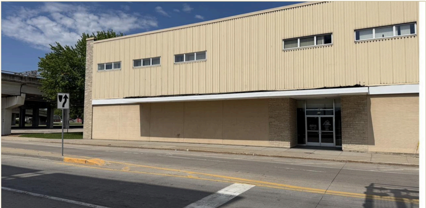
STREETWALL LOOKING NORTH ALONG S. BROADWAY TOWARD THE MASON STREET VIADUCT
