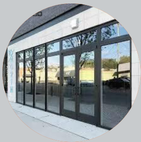
Exterior Loaded Entry
