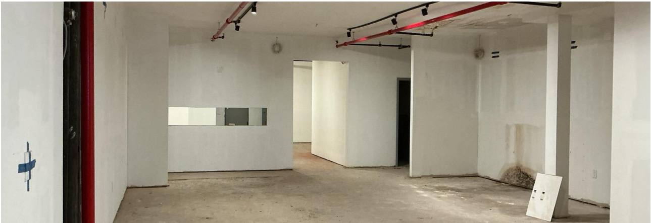
Shell condition — open layout, concrete floors, exposed sprinkler system, track lighting
