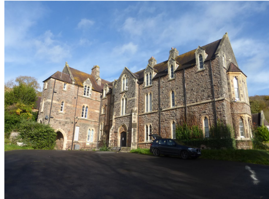
St Michaels, Cheddar Road, Axbridge, Somerset BS26 2DW
