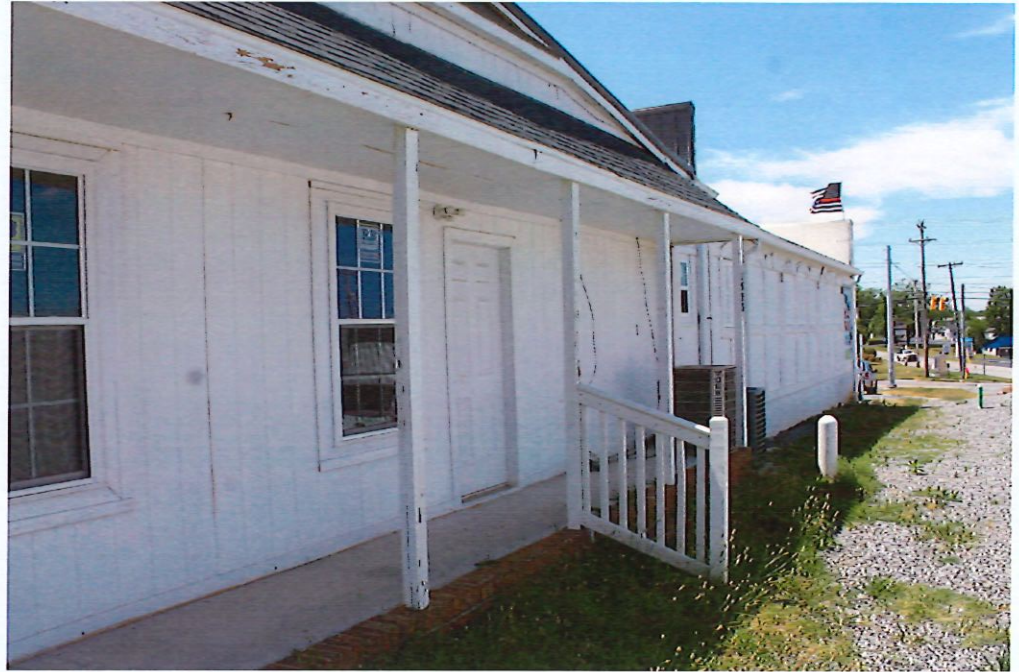
Side entrance to office area.
