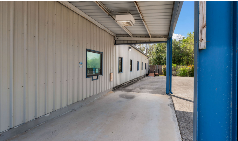
Covered exterior walkway
