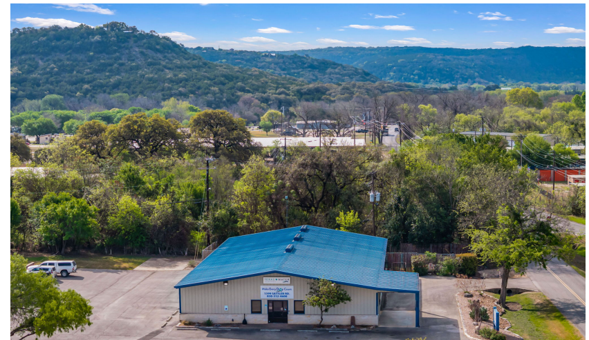
Aerial view of the property
