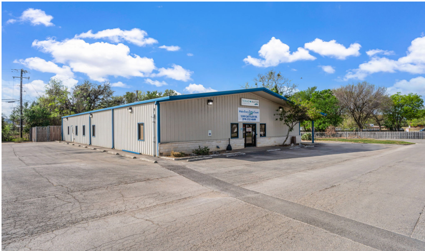
Exterior view of 1399 Sattler Road
