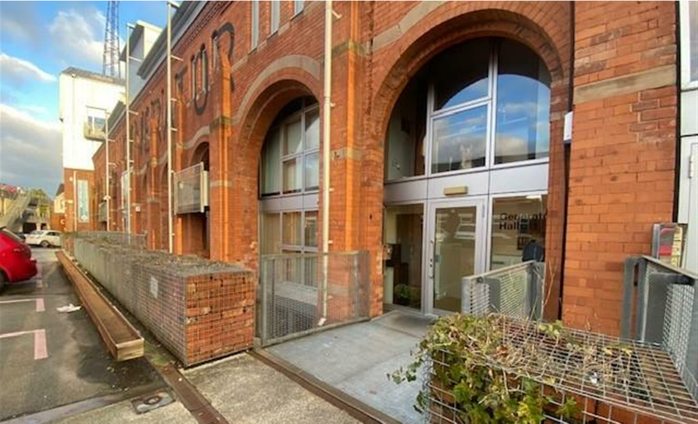
Units at Generator Hall, Electric Wharf, Coventry, CV1
